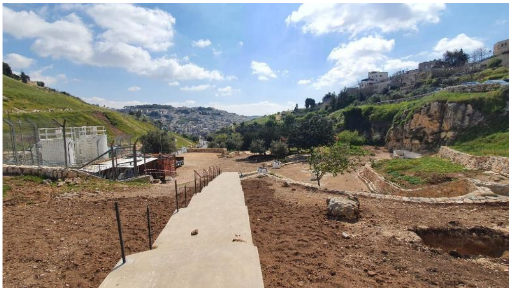
Works in progress on the Center for Ancient Agriculture
