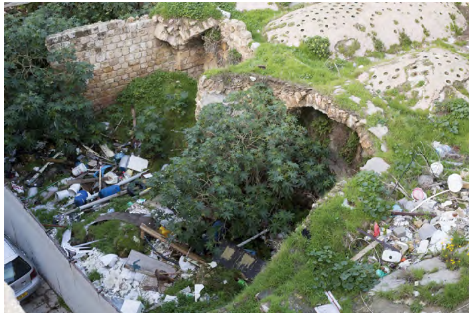
The small bathhouse (Hamam) neglected and partially destroyed.
