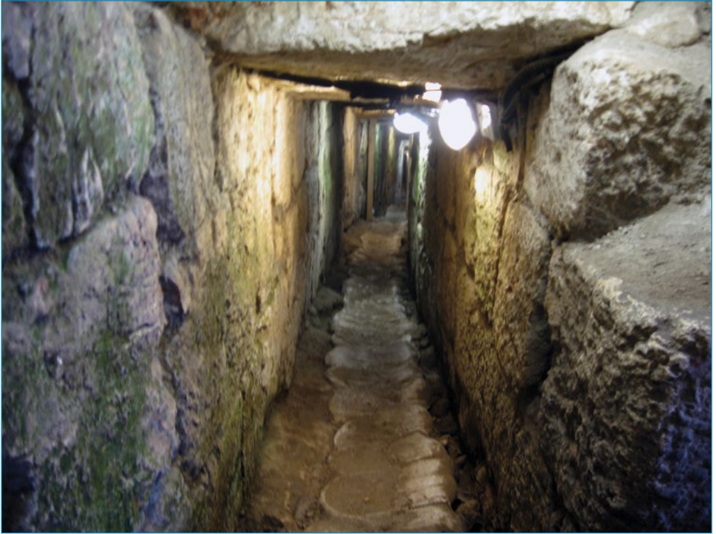
Tunnel underneath the village of Silwan
