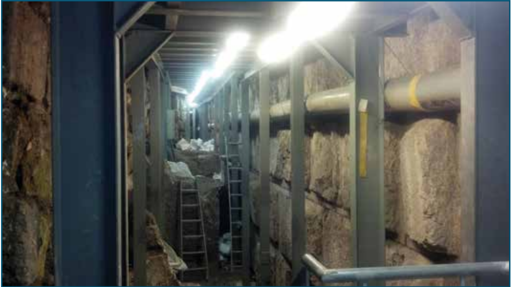
Tunnel underneath the Davidson Center
