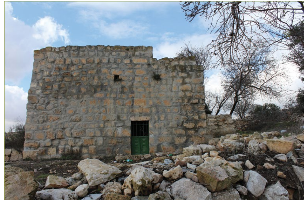
The renovated mosque
