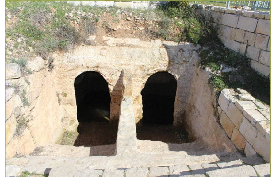
A cistern/ritual bath and the steps leading down to the two entrance points
