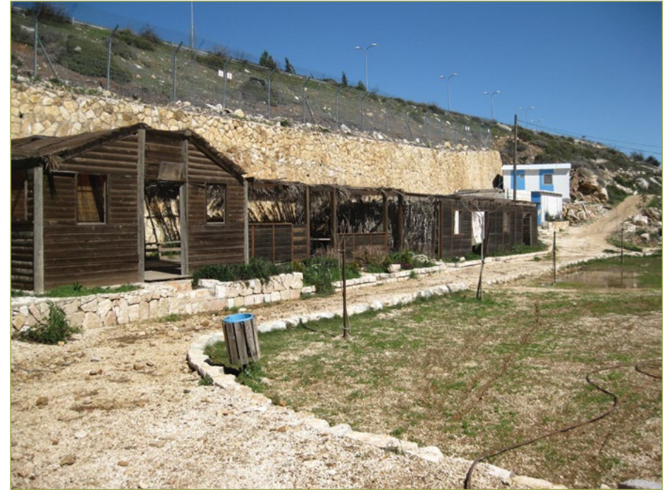
Ein Biyar – the entrance point to the shaft and the subterranean canal
