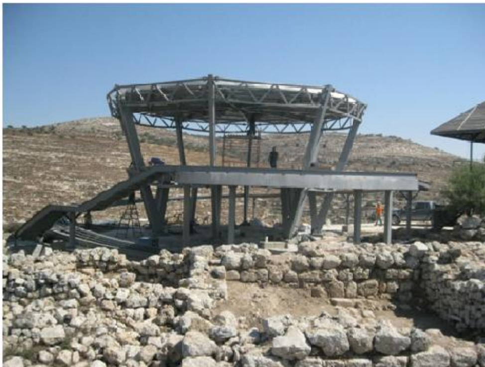
The Migdal Ha-Ro'eh Tower during construction
