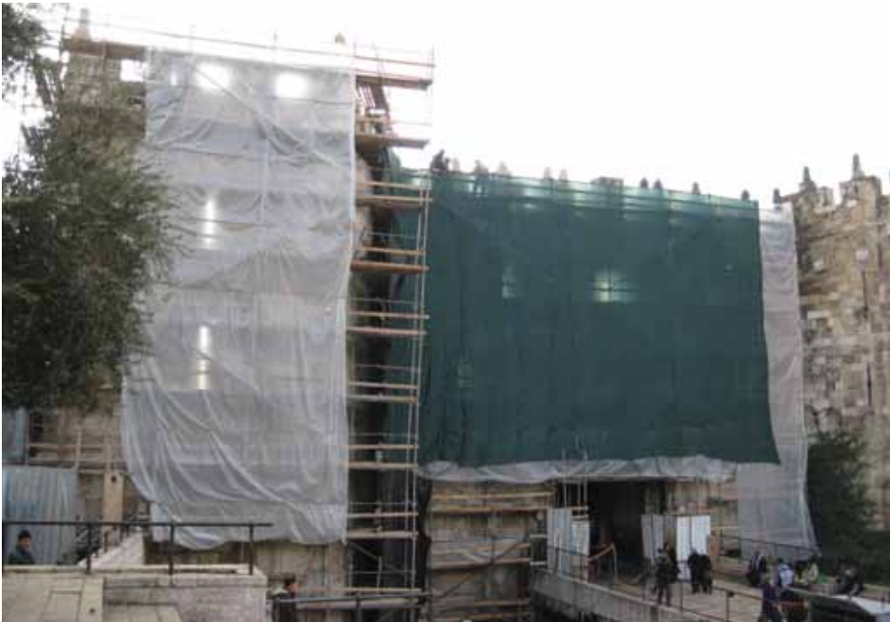
Damascus Gate/Bab Al-Amud preservation work 2011
