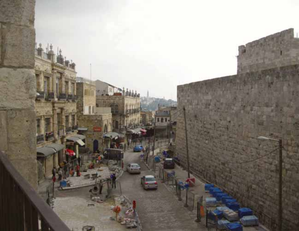
Construction works near Jaffa gate
