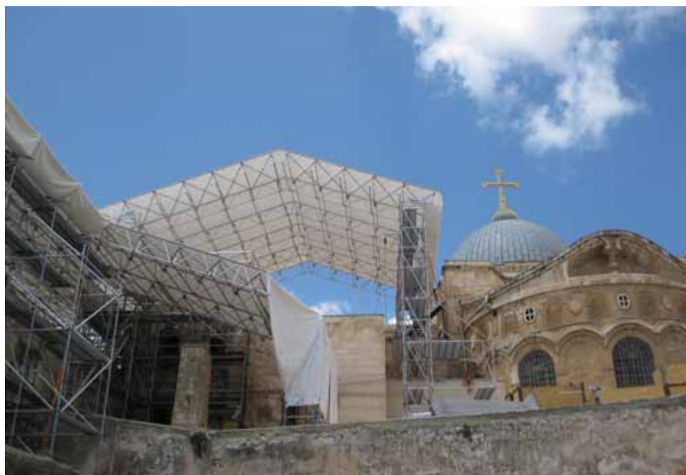
Renovations at the Church of the Holy Sepulcher
