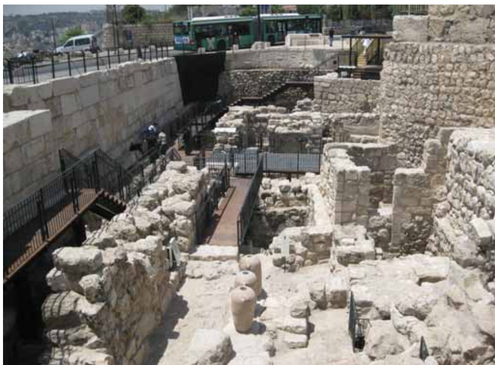
The Ophel walls in the Davidson Center after preservation works
